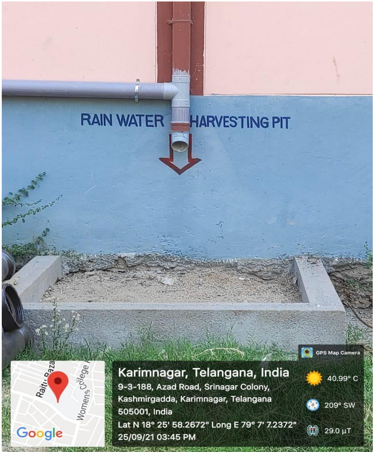
Rain water harvesting pit 02
