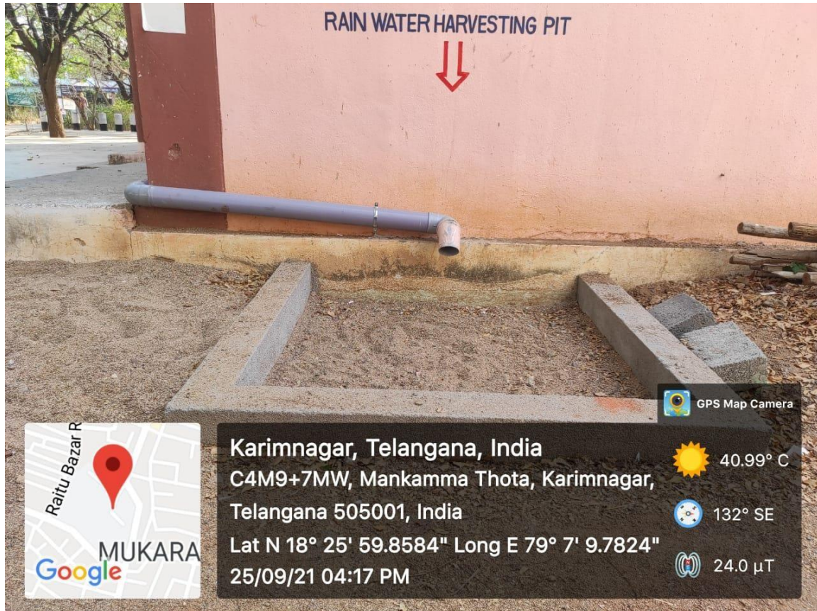
Rain water harvesting pit 01
