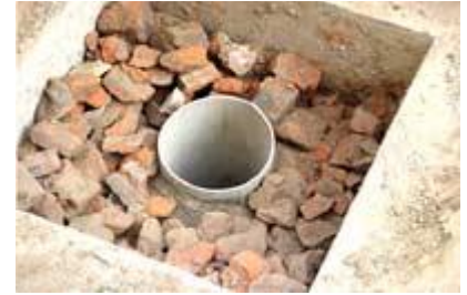
Filter materials in a soakaway
