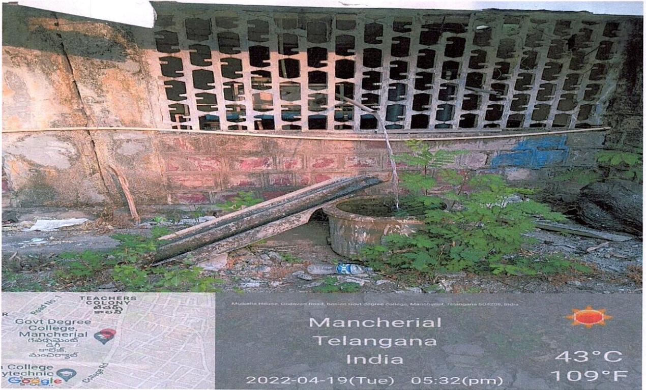
R. O Plant waste water
