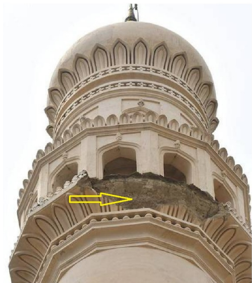
Fig. 3 The minaret of over 425-years old Charminar from where a huge chunk of plaster ( 2.5 \times 0.8 \text{ m}^2 shown by arrow) fell down on May 1, 2019 (adapted from The Hindu, May 3, 2019).
