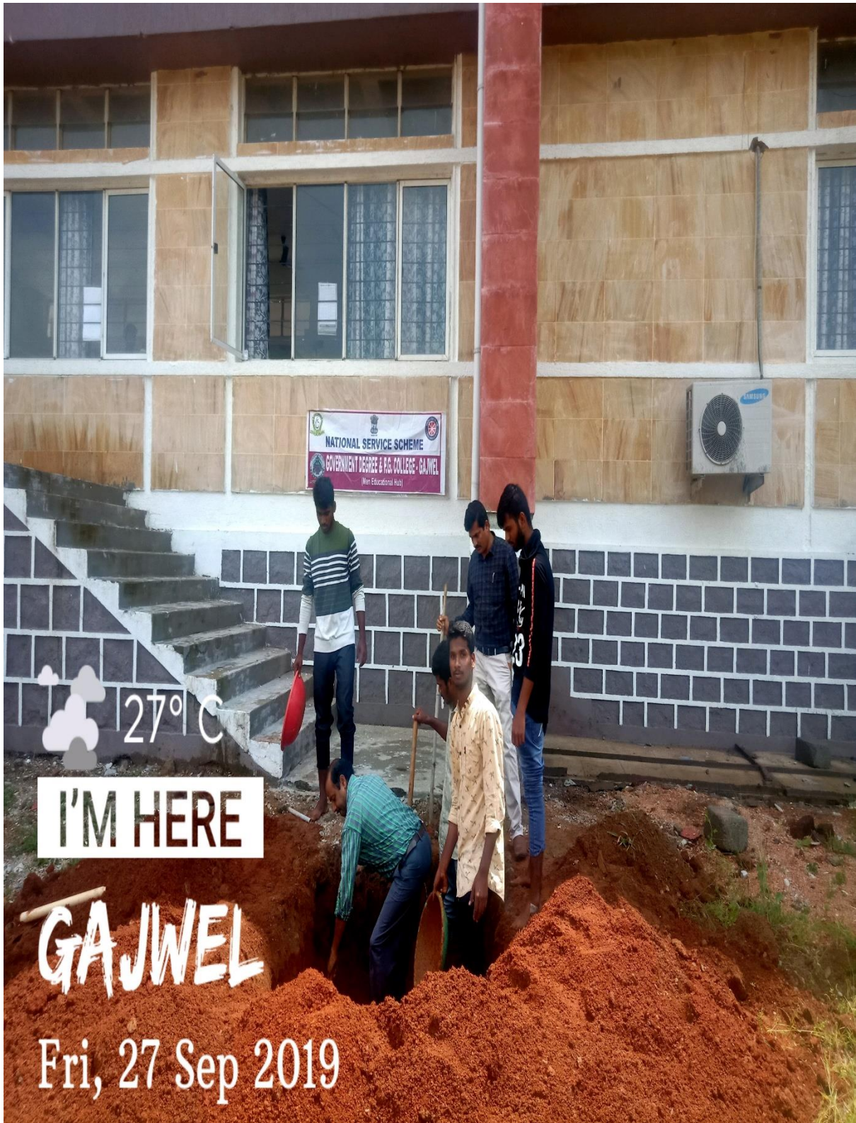
NSS Volunteers digging a Rain Water Harvesting Pit-1
