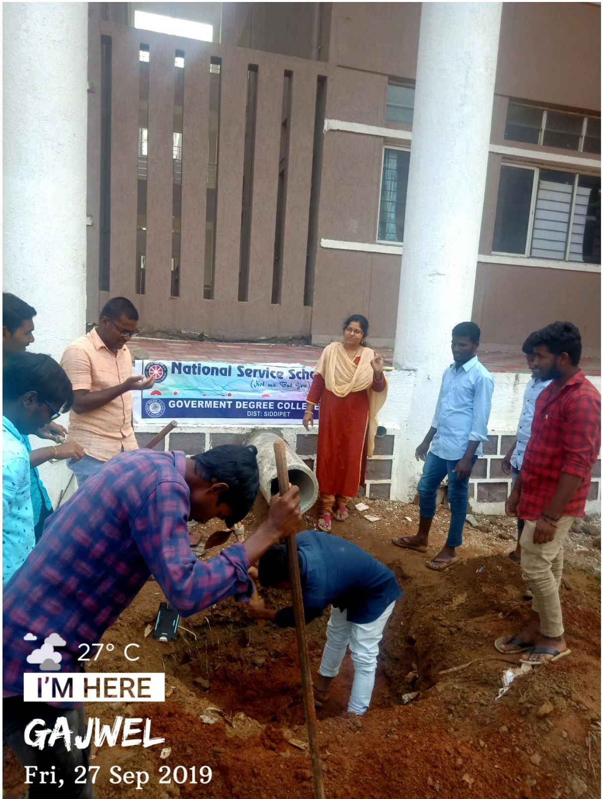
NSS Volunteers digging a Rain Water Harvesting Pit-2
