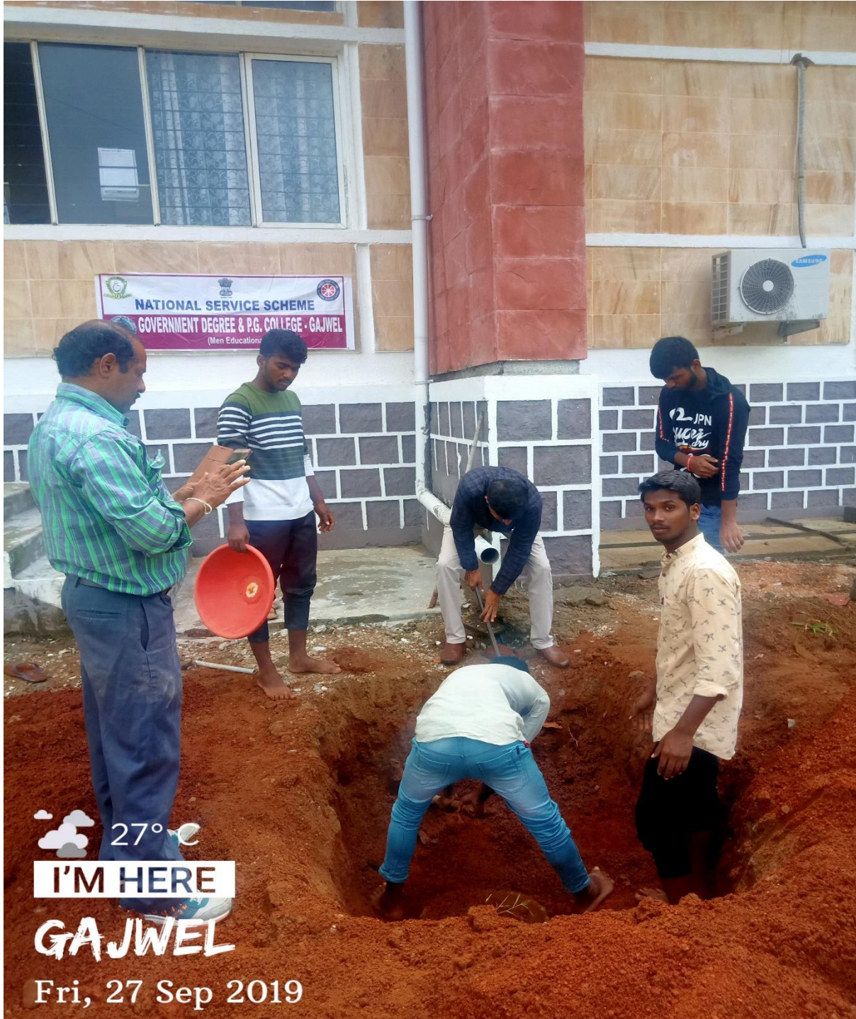
NSS Volunteers digging a Rain Water Harvesting Pit-1
