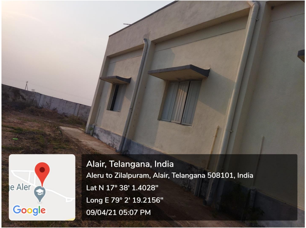
PVC pipes around the building to drain out the rain water
