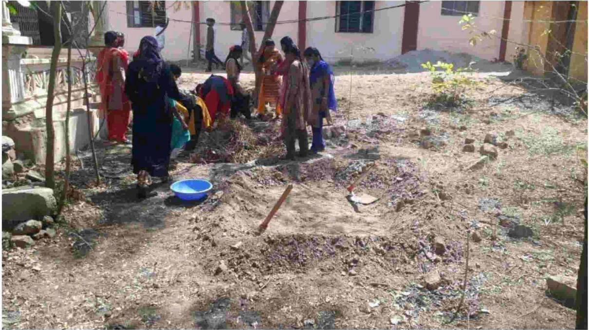
Old Cement sheets used for making Pit.
