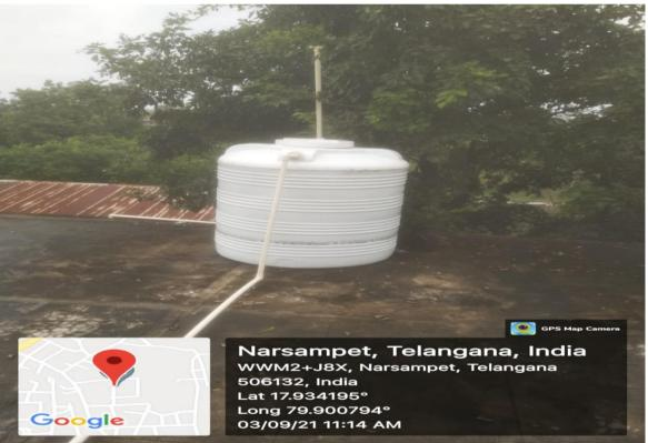
Newly Installed Over Head Tank on the Principals Chamber Roof for the water supply to the Principals Office & Haritha Haram Plants.
