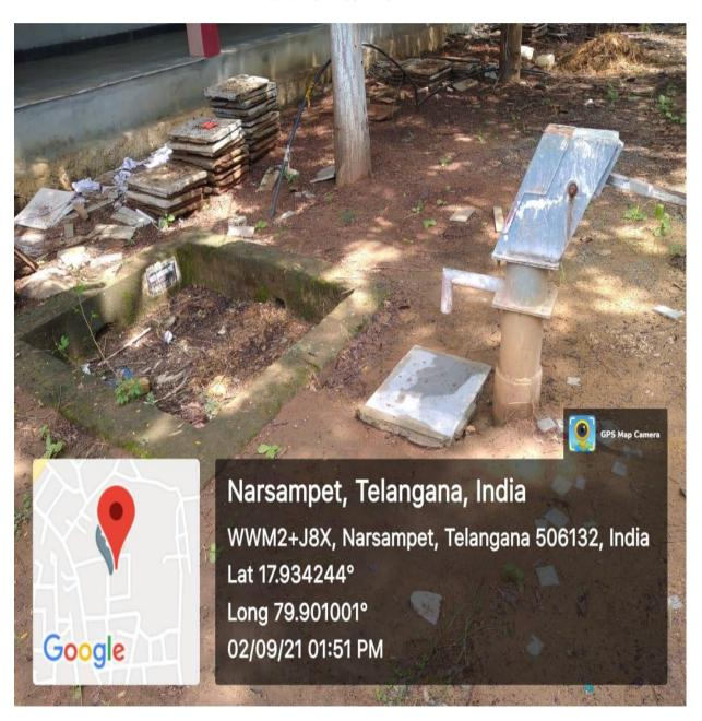
Water harvesting / Recharging pit was dug near the Hand pump. Date:-02-09-2021.
