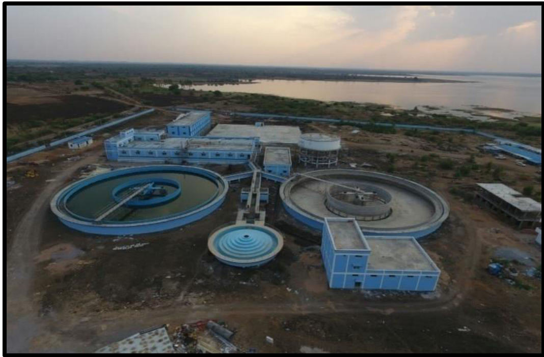
Structure showing WTP, OHBR and pump house
