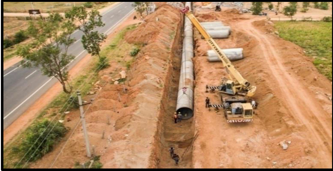
Laying of MS pipeline, Yellore segment in progress
