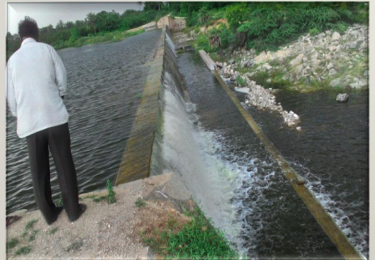
After Restoration of Weir
