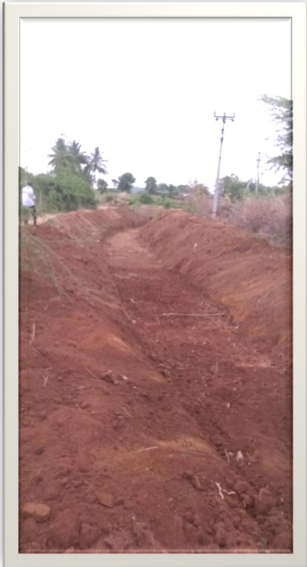
Feeder Channel After Restoration
