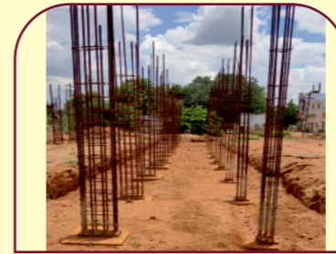
Construction of New Class Rooms
