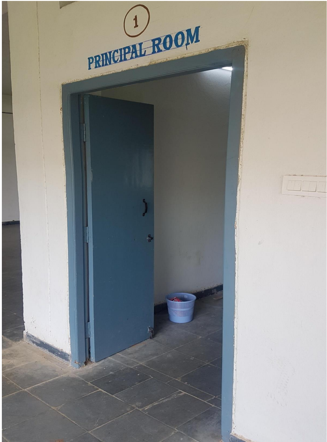
At principal chamber
