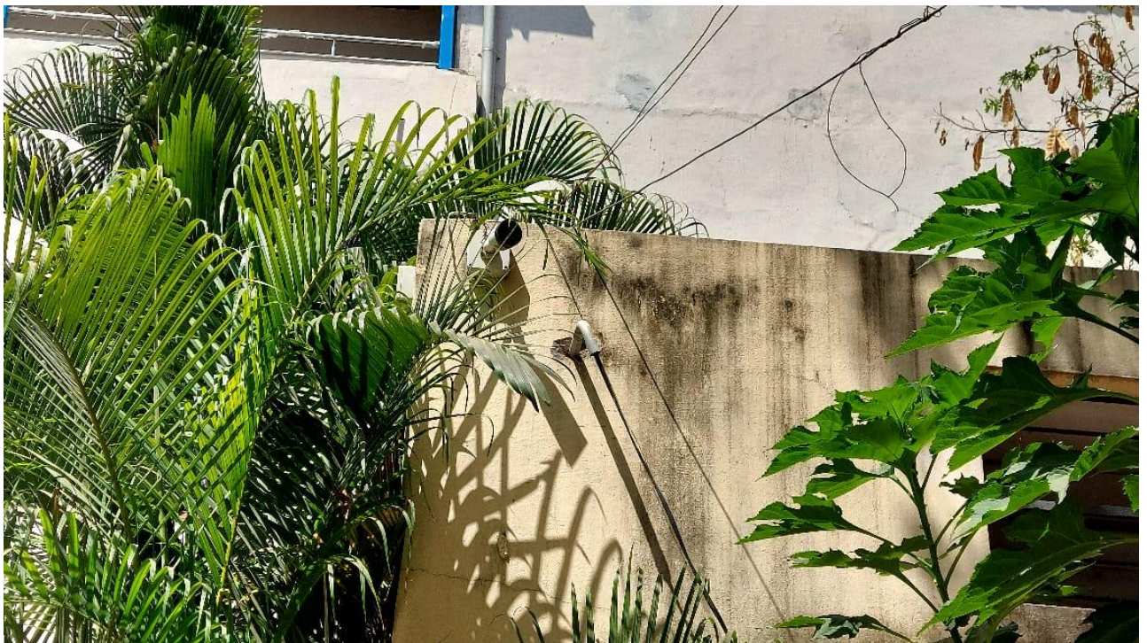
CCTV cameras installed in college campus
