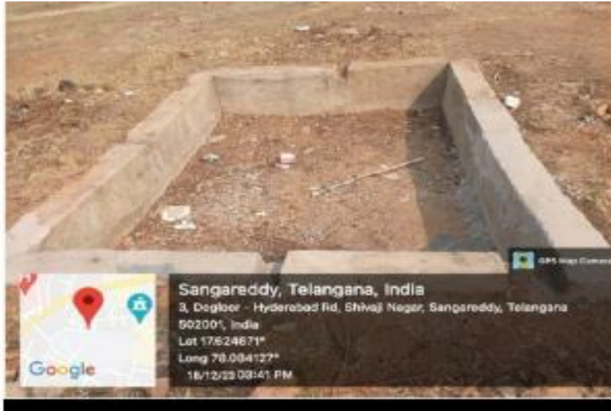
Water harvesting pits
