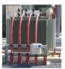
It is an underground WYE or delta-connected system used to provide a ground path or neutral in a three-phase electric power system. This can help reduce the voltage transients when a ground fault happens.
