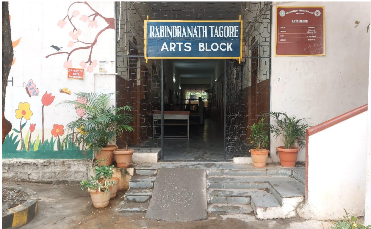
Ramp Facility at Arts block
