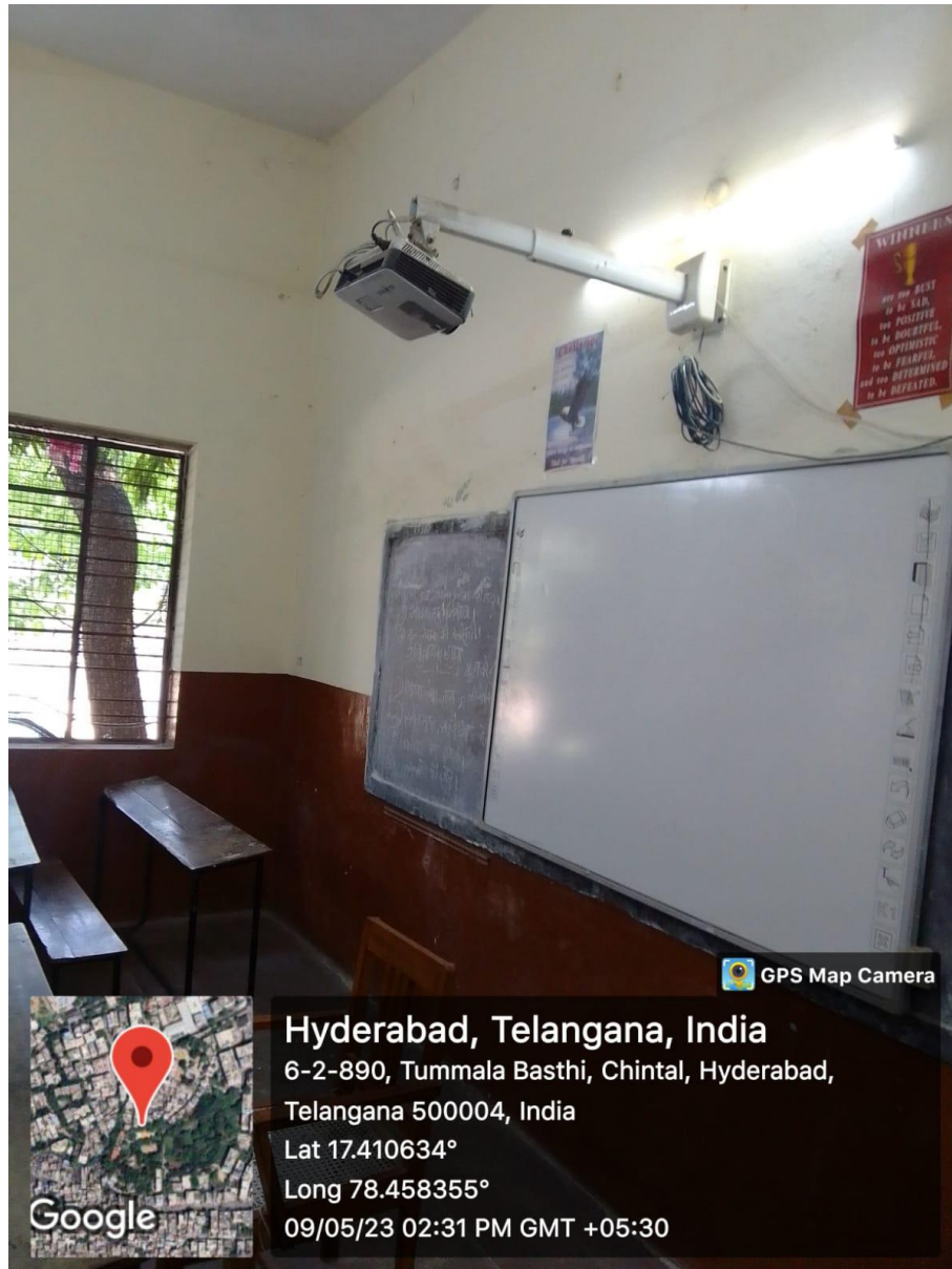
ICT facility in in Room No .4
