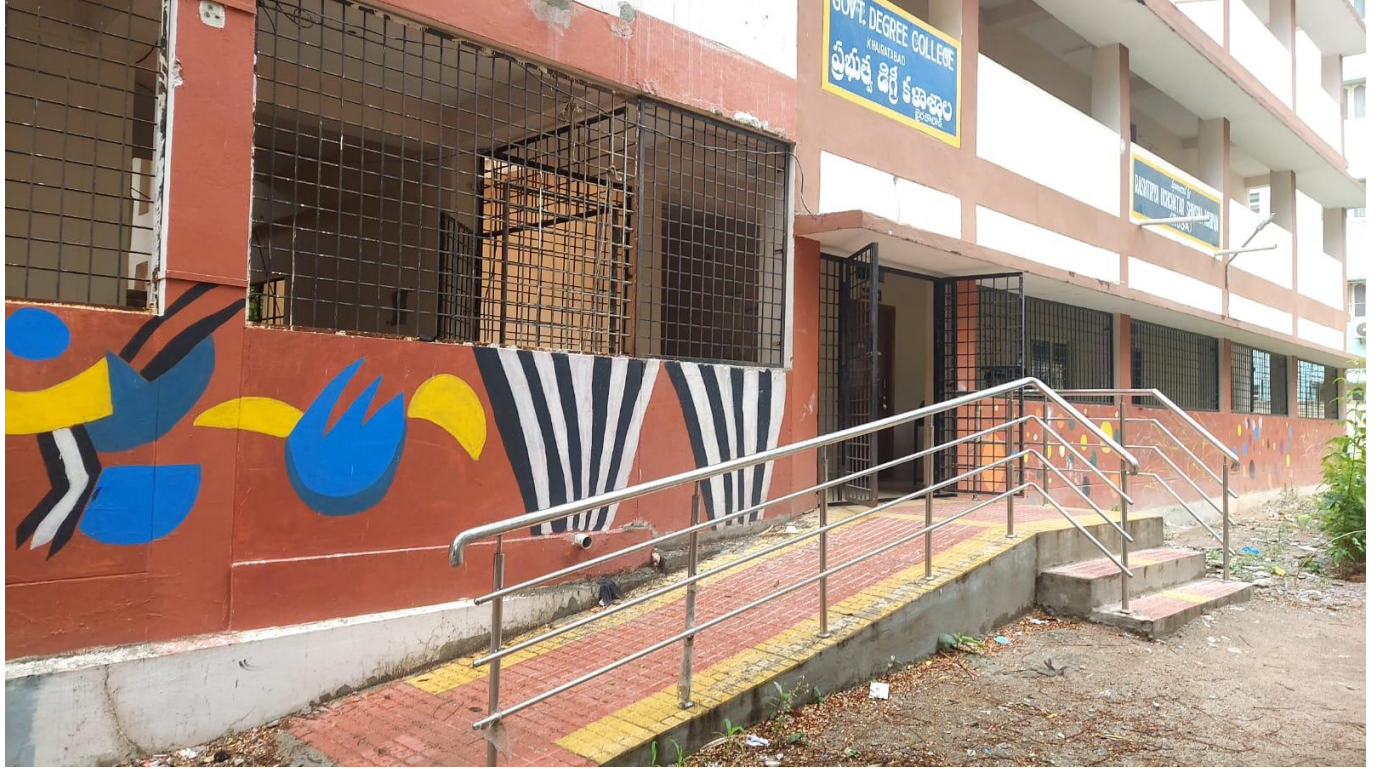
Ramp Facility at commerce block
