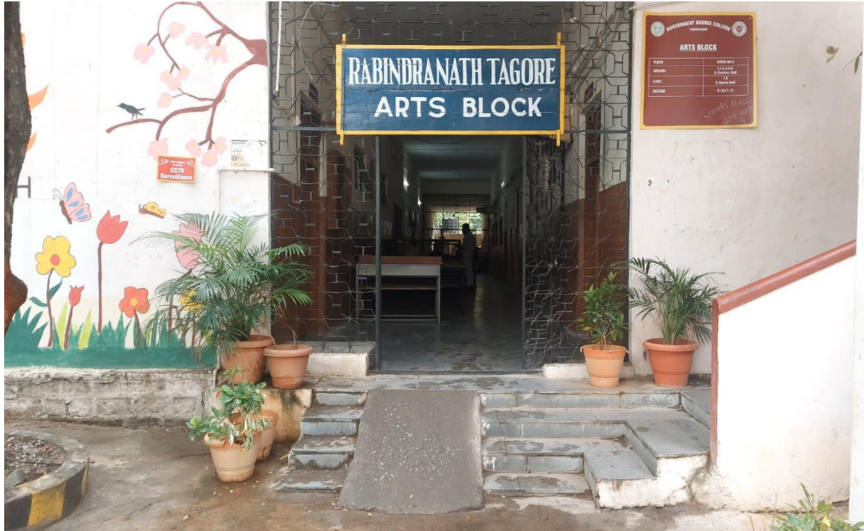
Ramp Facility at Arts block
