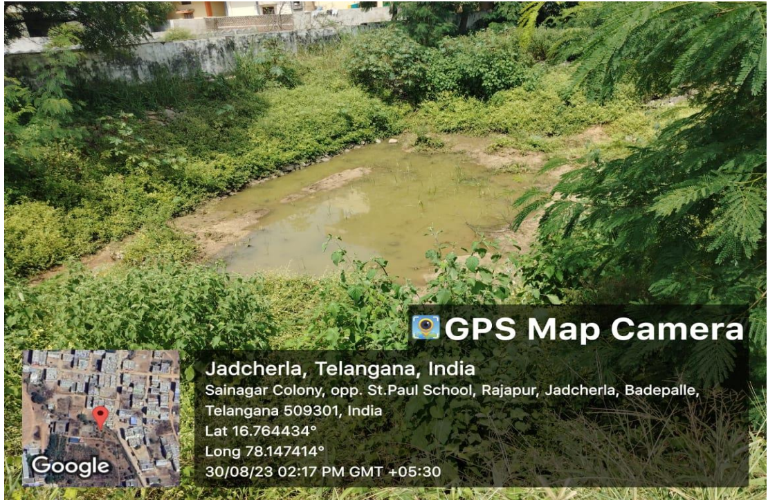
Rain Water Harvesting Pit
