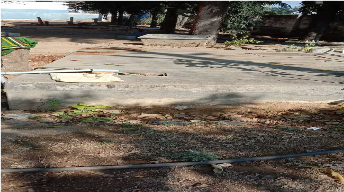
Tanks are build in campus for water needs
