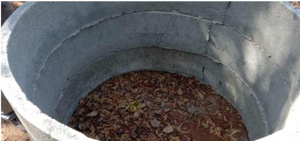
Solid waste recycling pit
