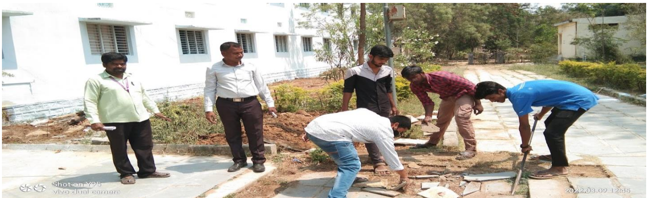
3 Days Special Camp (Day - 2: 09.03.2022): Pavement Repair in between A & E Blocks
