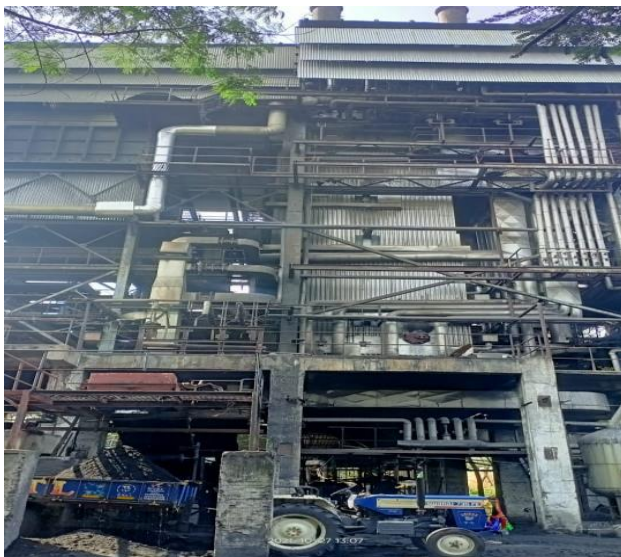
SHALIVAHANA GREEN POWER LTD. 6 MW BIO POWER PLANT MANCHERIAL
