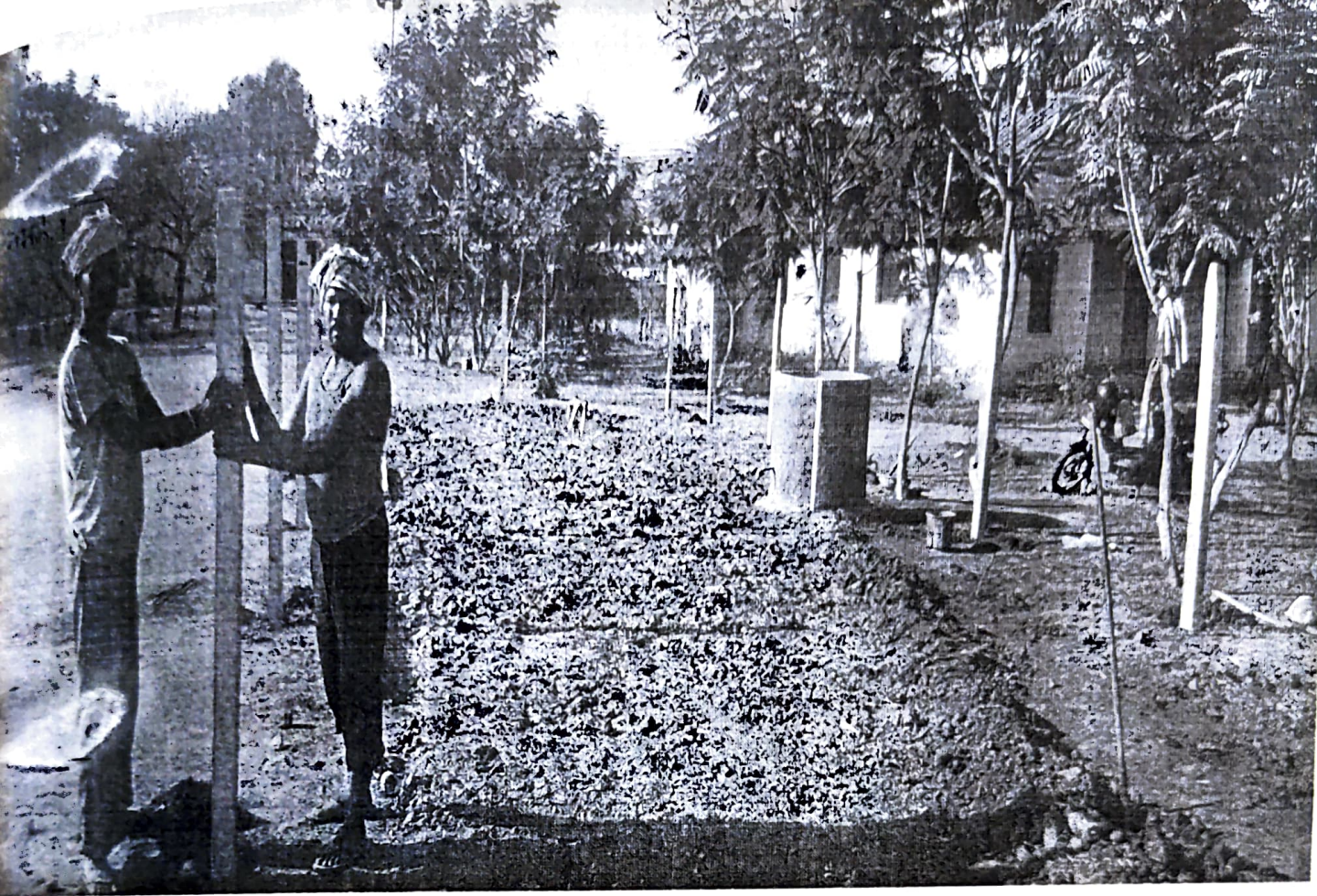
Installing the cement poles for fencing the garden.
