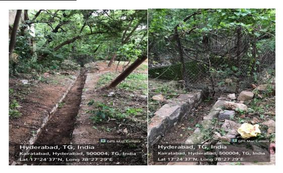
Water conservation isplanned by diverting the spilled water from the drinking water dispensers through an aqueduct to percolate into Rain water harvesting pit.
