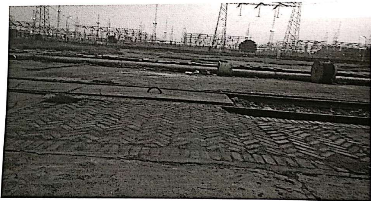
Power Station at National Thermal Power Corporation
