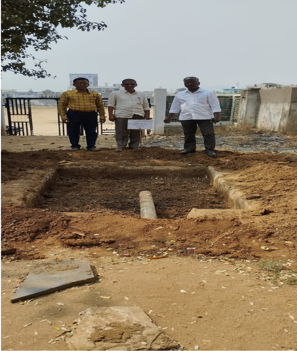
Principal inspecting the work of digging pit
