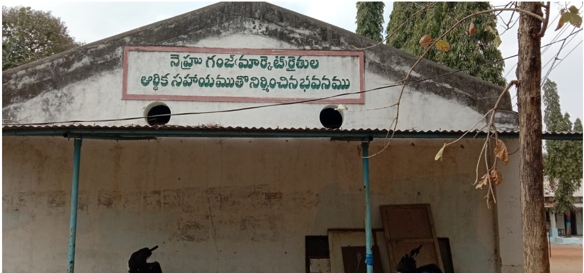
A space for vehicles parking was built with the assistance of others
