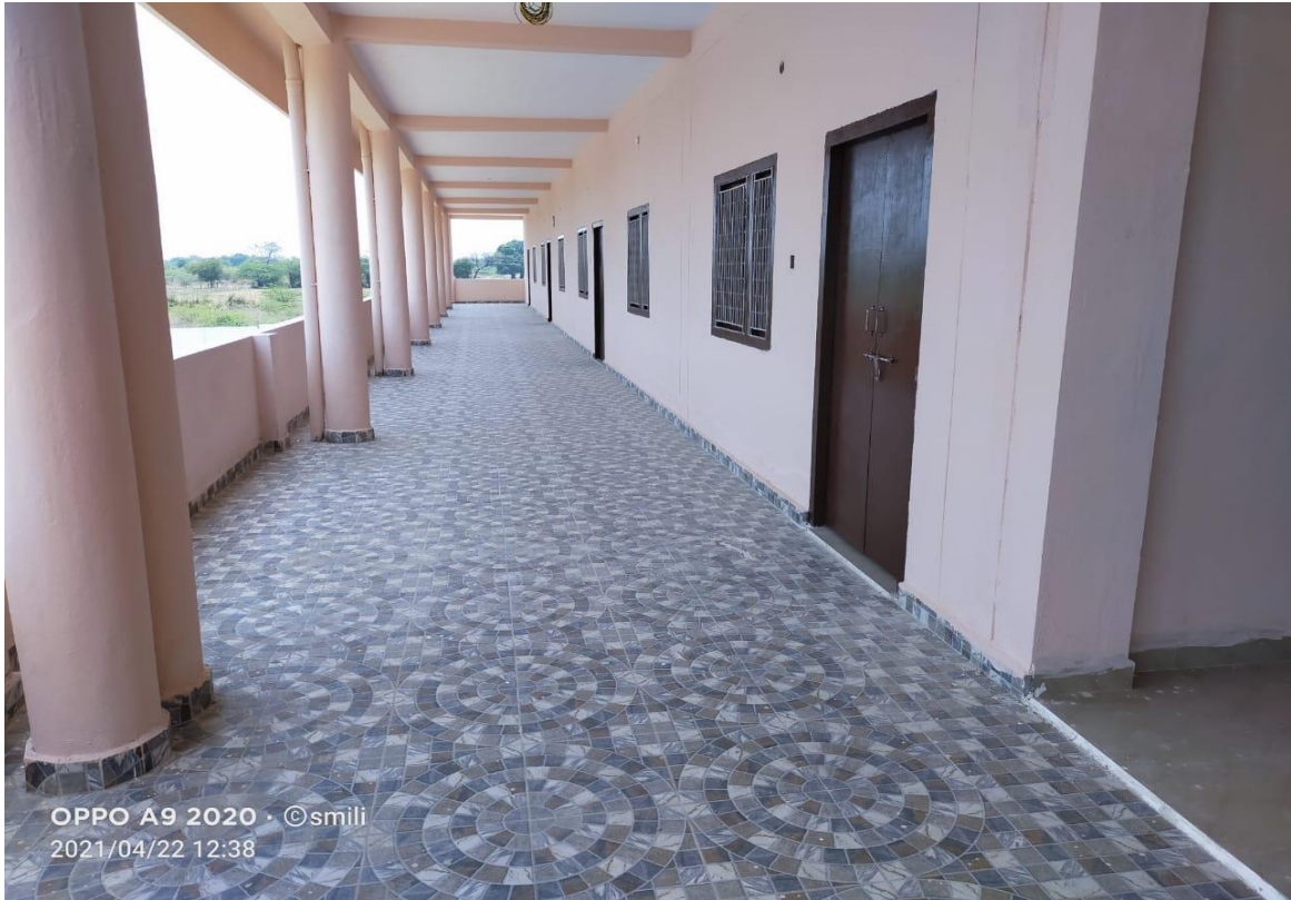
BULIDING LEFT CORRIDOR
