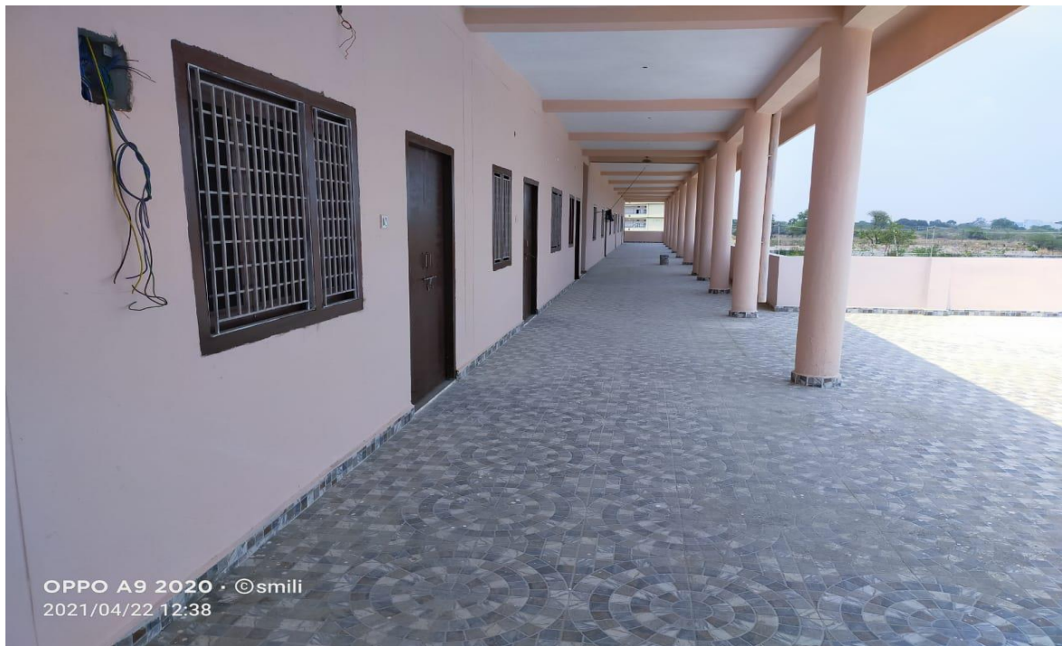
BULIDING RIGHT CORRIDOR
