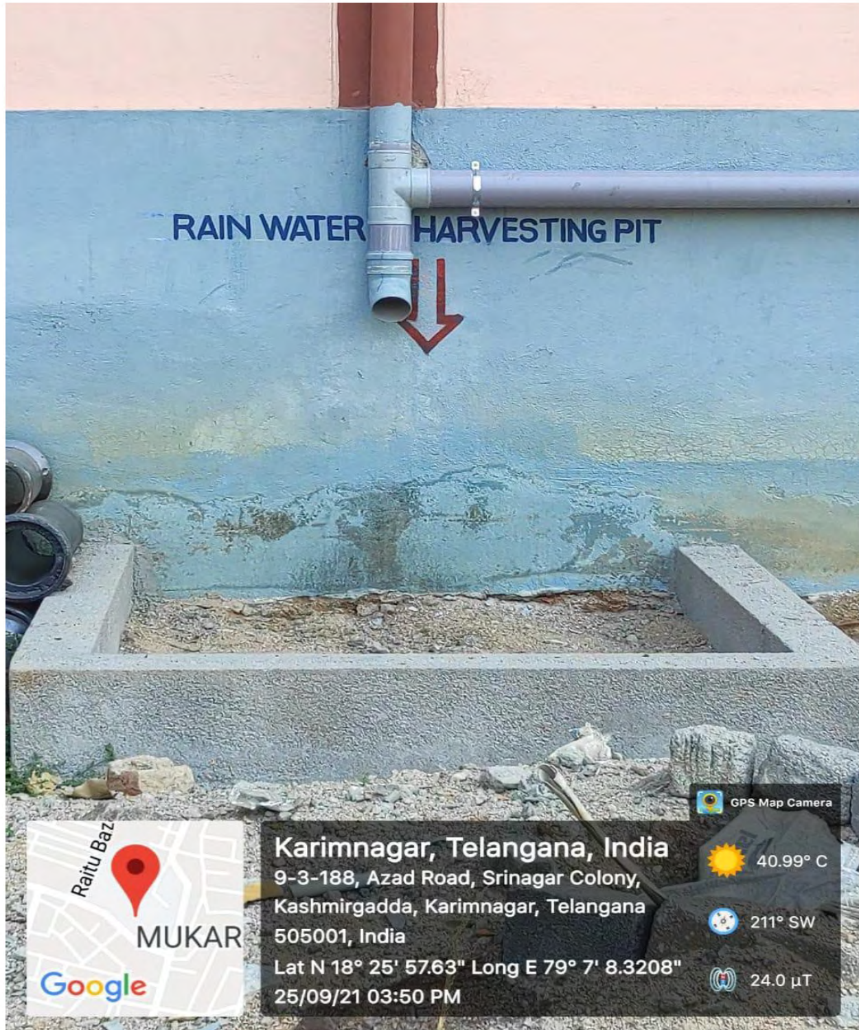
Rain water harvesting pit 03
