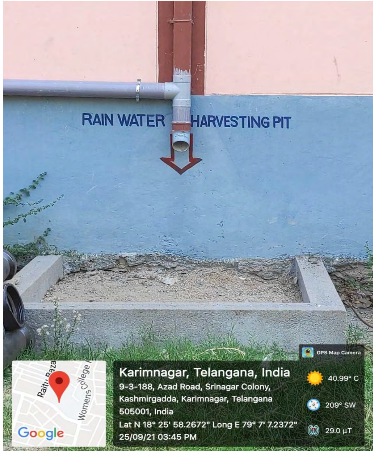
Rain water harvesting pit 02
