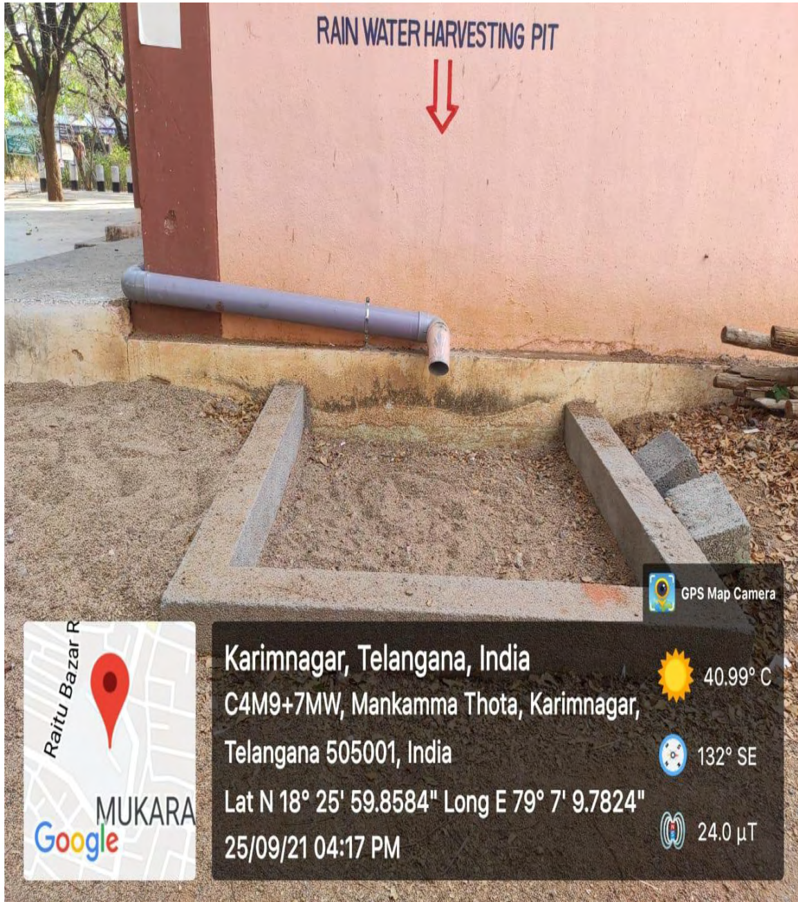
Rain water harvesting pit 01
