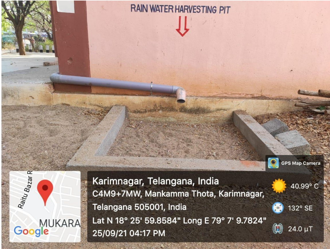
Rain water harvesting pit 01
